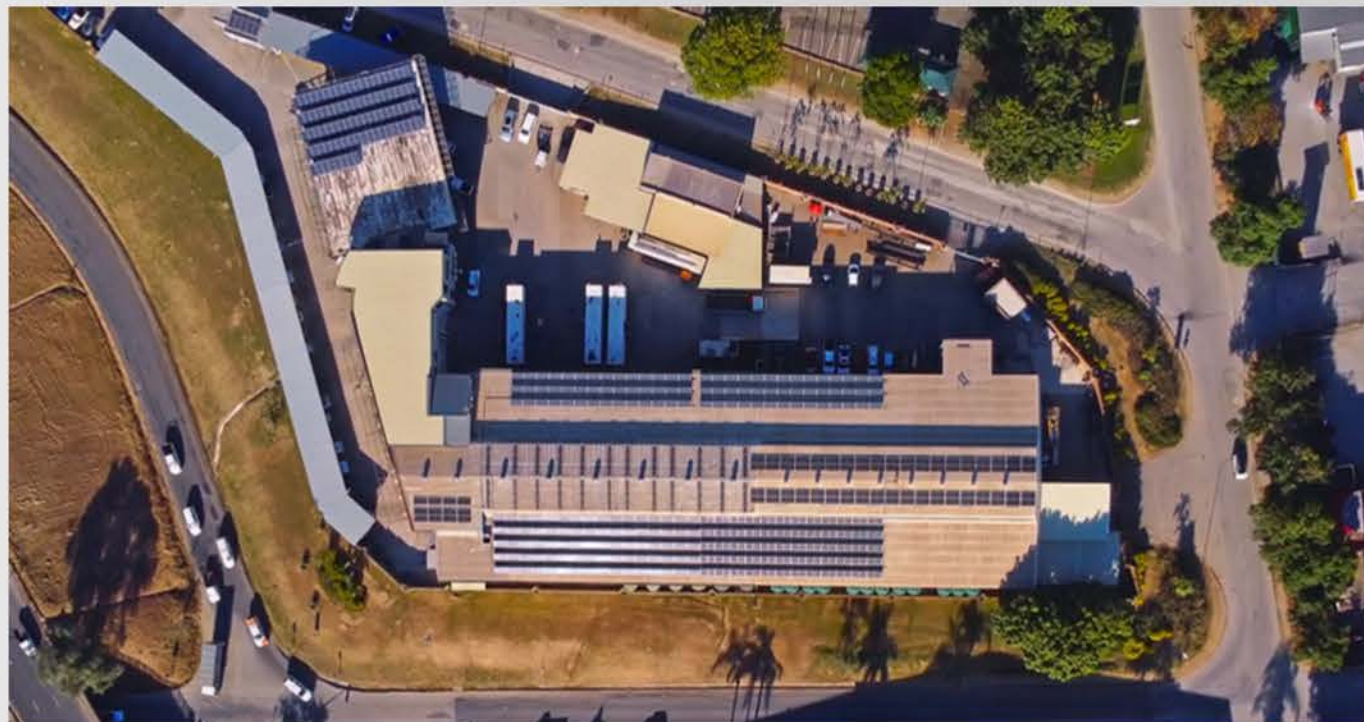
(Nelspruit, Mpumalanga Head Office arial image)
